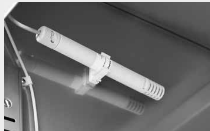
Humidity control kit inside the room with electronic probe for detecting relative humidity with maximum precision.
